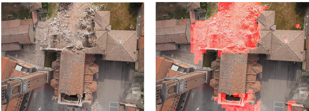
Figure 9. UAV image taken after the 2012 Mirabello earthquake (left); damaged regions mapped by our method in red mask (right)
